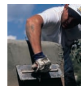
3. Making sure the mesh is fully covered by the base-coat
