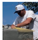
2. Embedding mesh to keep the repair strong and long-lasting
