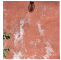
Efflorescence/Chalking
